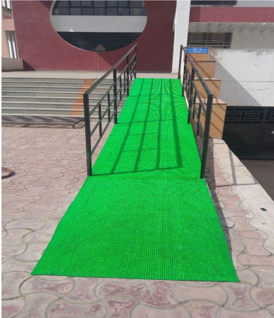
Ramp / Rails for Divyangjan (To Parking Area as well as Upstairs - Easy movement and access to all acilities)
